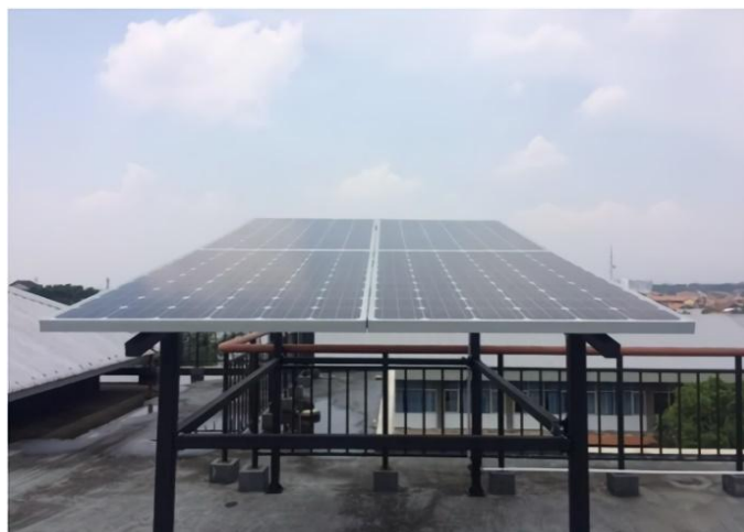
Fig. 1. Installation of 1 kWp at ITENAS Bandung
