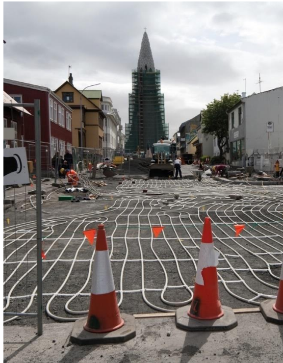
Fig.2. Road heating with wastewater to avoid icing, and ice formation
