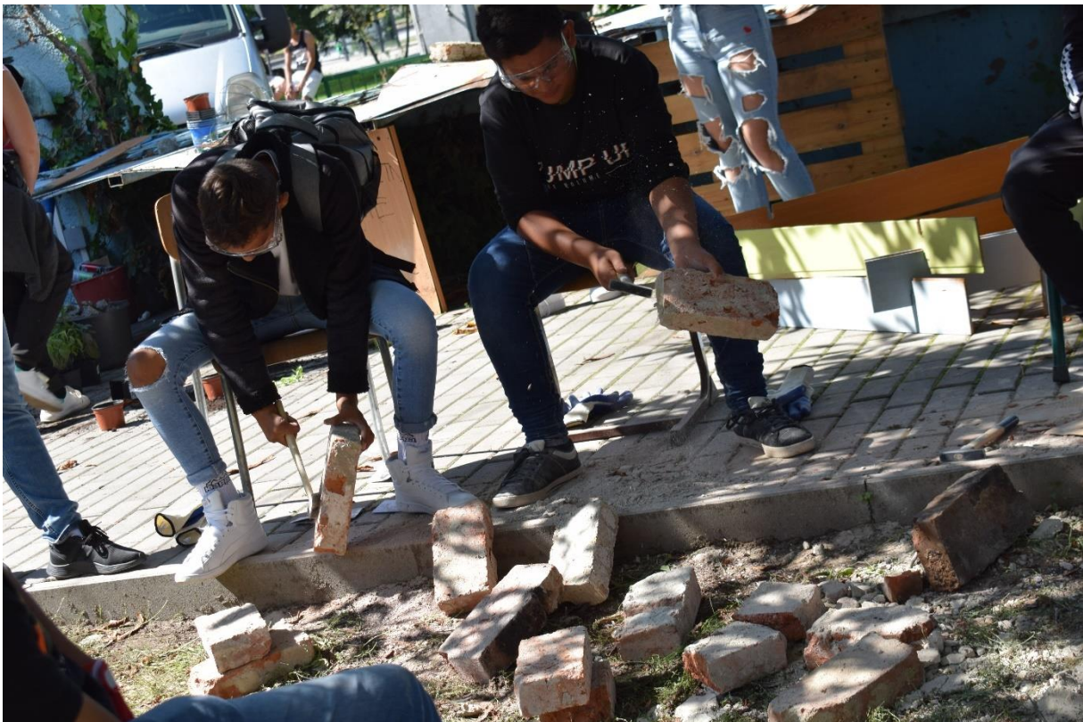
Figure 35. Dr. Ámbédkar students are preparing the brick for building the raised bed. Photo by Anita Reith
