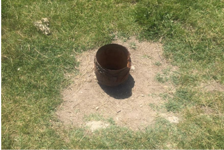
Figure 3: Plugged geothermal well, as a possible energy source Source: Own research, Biharnagybajom, 2020
