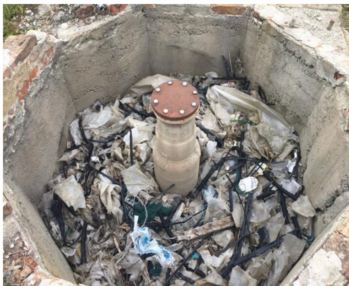
Figure 2: Closed geothermal well, as a possible energy source Source: Own research, Biharnagybajom, 2020
