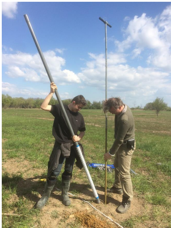
The installation of a groundwater well.
